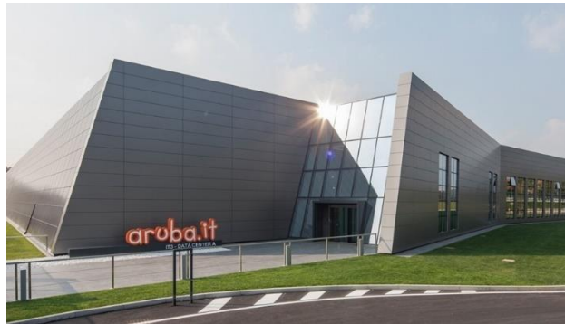
Figure 5: Euronex Data Centre in Bergamo, Italy
