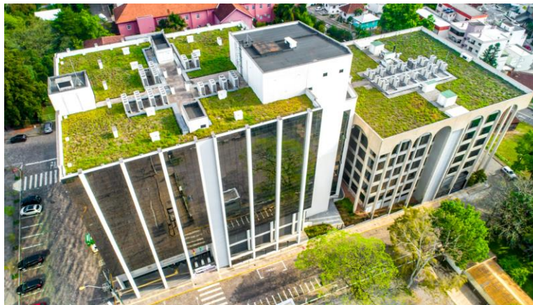
Figure 8: Example of green roofs. Source:
