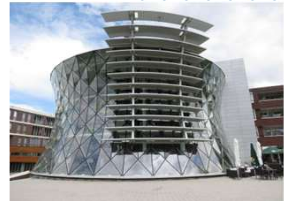
The energy station is situated in the basement of the Heerlerheide Centrum (HHC) Picture: Sciencedirect
